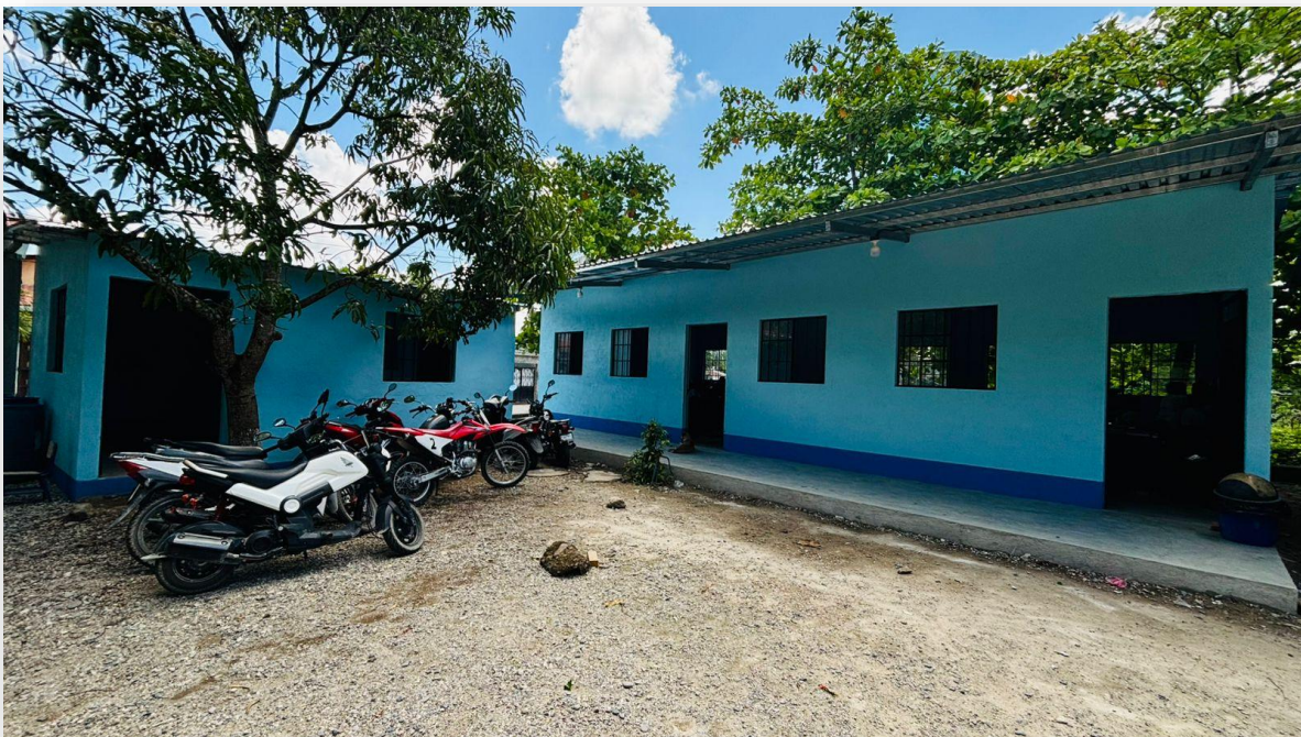
Photo of the exterior of the new classrooms, with painted finishes.
